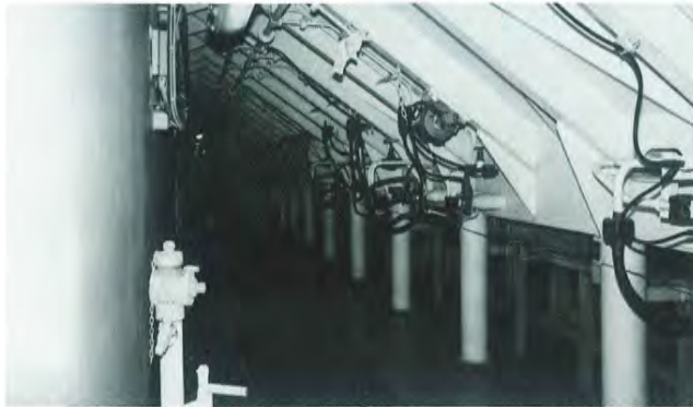
Global Design Series vibrators are used to enhance material flow in large structures, such as this self-unloading cargo ship.
